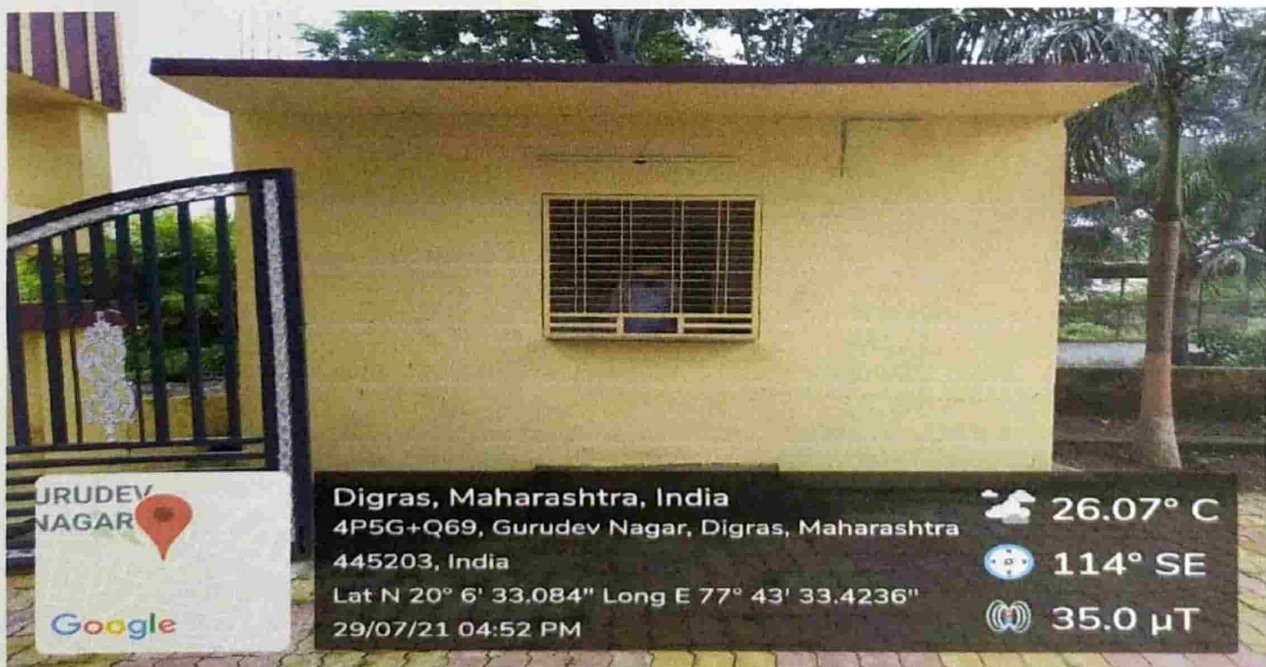
College Main Gate and Security Guard Room
